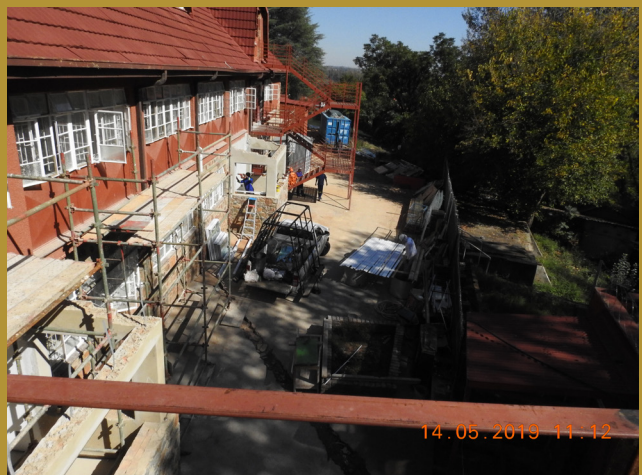
External replacements including window repairs, plastering, etc.
